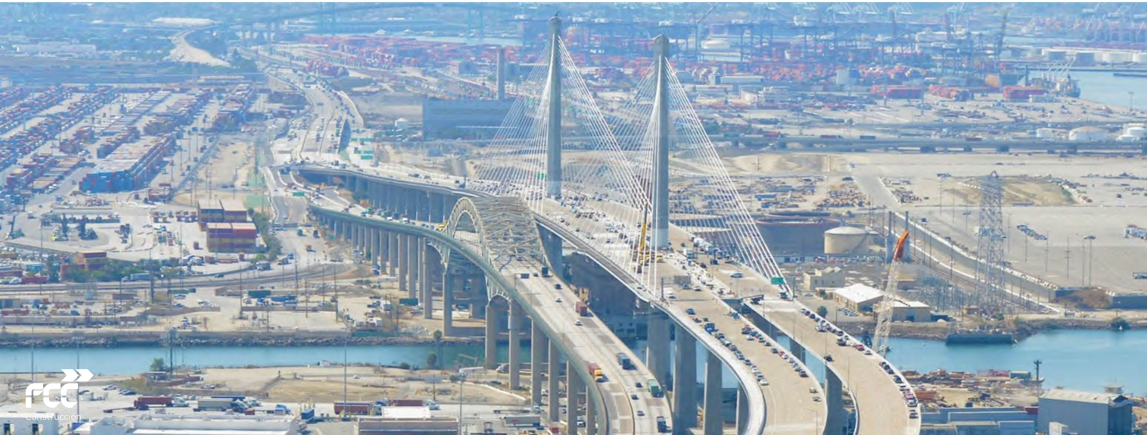
Gerald Desmond Bridge, United States
